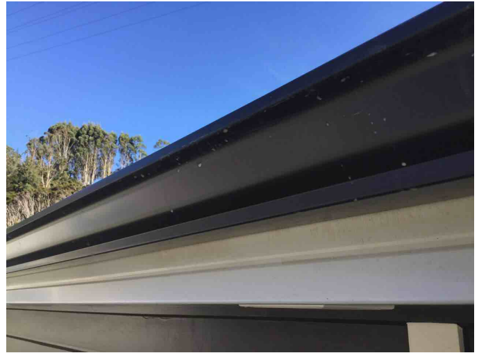
Metal spouting system and pressed metal fascia. These systems are generally low maintenance and robust. Recommend washing at least twice yearly to remove grime build up which slowly deteriorates the paint coat.
