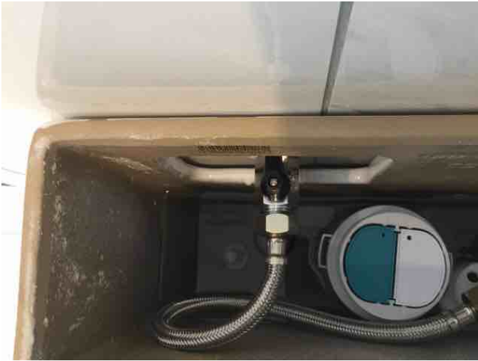
Toilet cistern has an isolation valve. Good detailing.
