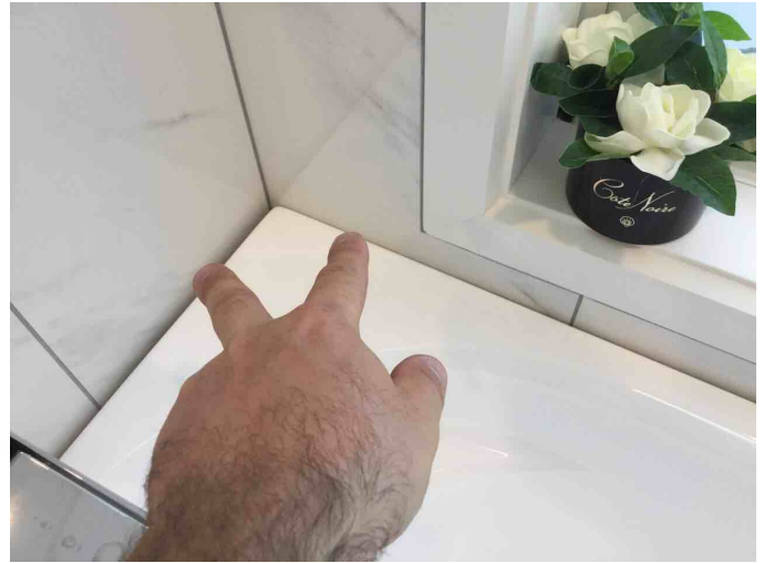
In the bath is left in situ, consideration should be given to sealing the bath against the tile to prevent water being slashed over the back lip. There is now access for mopping or cleaning.
