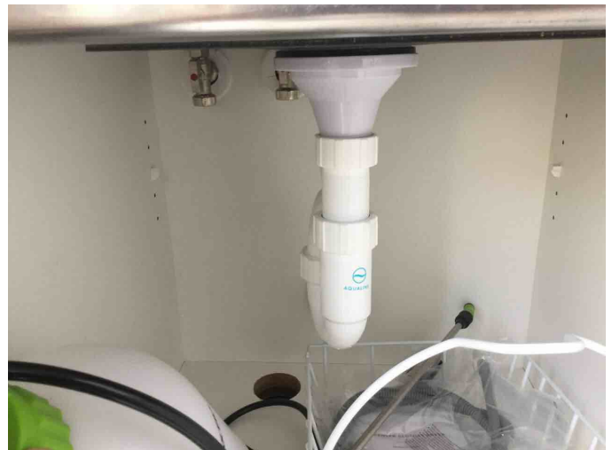
Washing machine not currently plumbed in. The Tub plumbing tested ok, no concerns sighted to the plumbing, connected to the tub, within the cupboard space.
