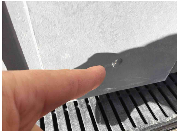
Noted. Slight popped fixing. Mainly cosmetic, no significant concerns. Small remedial required.
