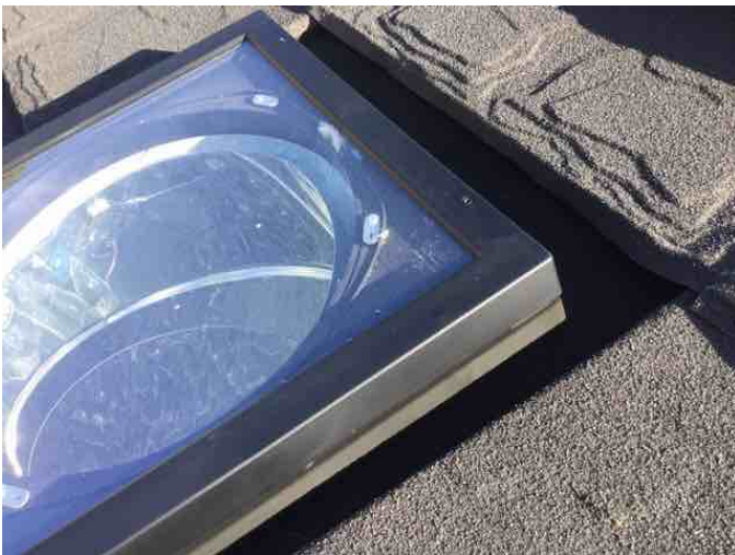
Anually inspect all penetrations. Potential debris build up, behind the flashings can cause moisture ingress. No concerns sighted.
