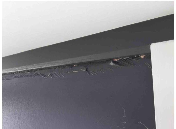
The paintcoat has significant defects adapting the timber trim / soffits Remedial work is required to maintain the paint coat integrity.
