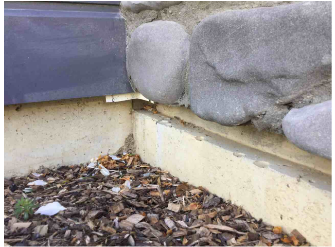
The perimeter of the foundation was sighted, no evidence of stress cracking or subsidence. No concerns.
