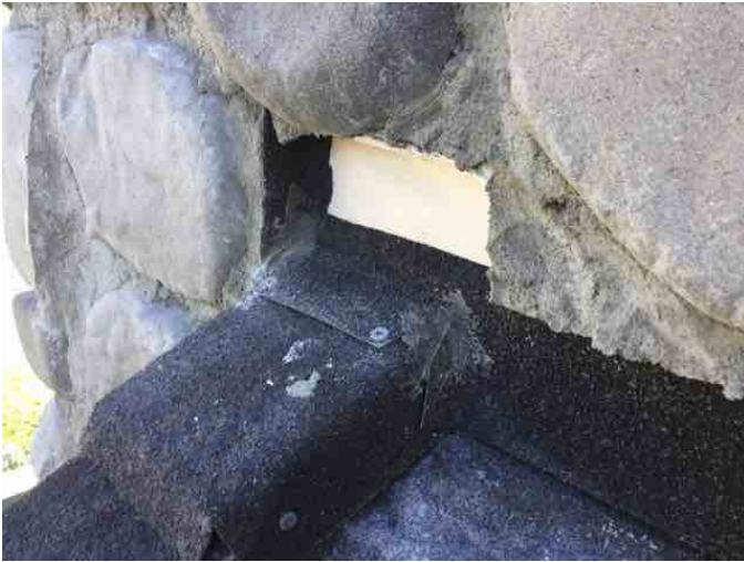
Example. Annually inspect all silicone seals around complex junctions.
