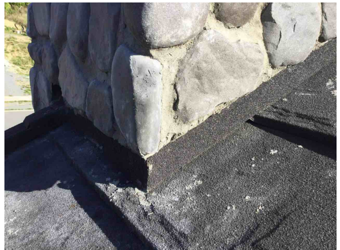
Dummy chimney flashing well detailed. No significant concerns. Mortar residue is evident on some of the roofing tiles.
