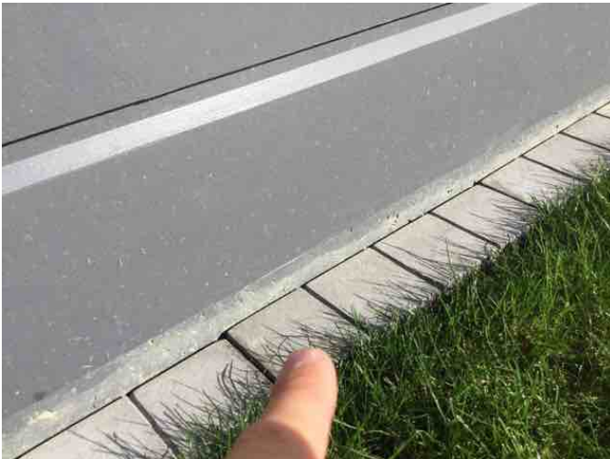
Consider mortaring the mowing strip in place.
