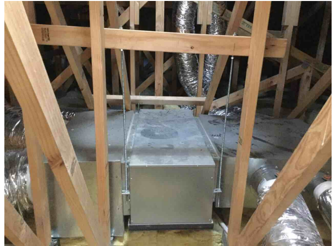
Significant ducted heatpump sighted. No concerns. Become familiar with any servicing, that may be required.
