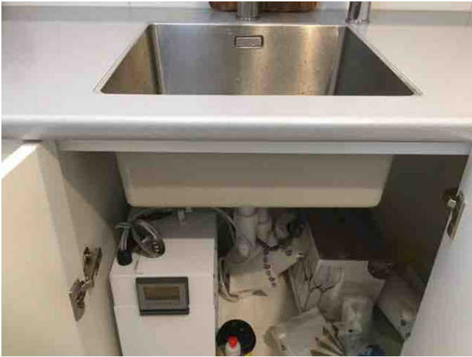
Butlers pantry. Well detailed no concerns. No concerns to pipe work and wastes under sink. Seperate undersink hotwater boiler unit noted.
