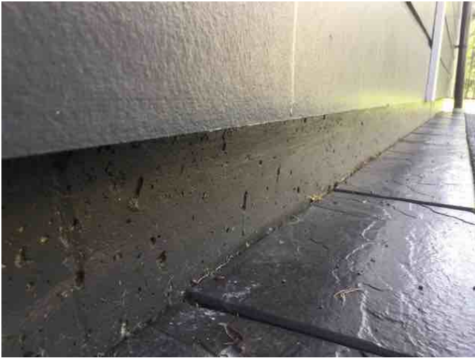
Engineered concrete ring and slab foundation. Commonly found in modern builds. No concerns sighted.
