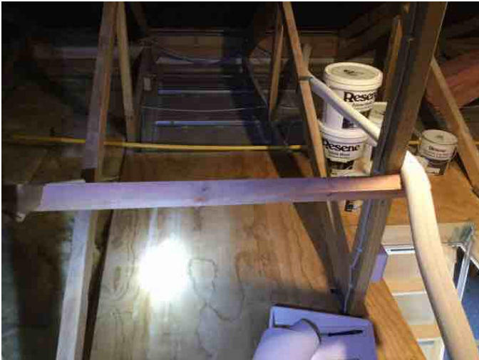
No insulation above the garage area. Not deemed a requirement by council.
