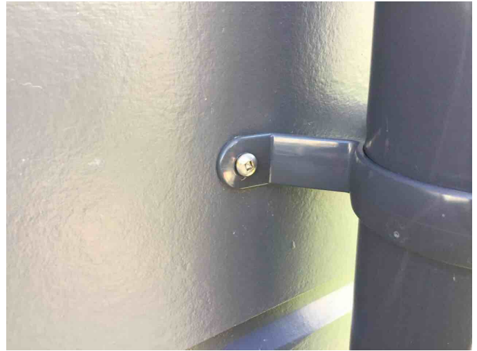
Noted stainless steel down pipe fixings have been used.
