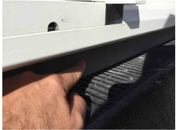
Noted. The section of cladding under the sliding aluminium door is floating, and could easily be knocked and broken. Recommend fixing it back to the foundation.
